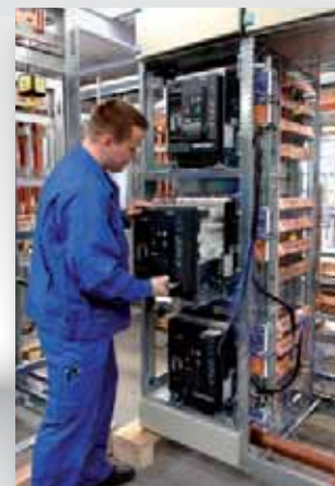
Assembly of a switch cabinet
