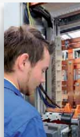
Assembly of a switch cabinet
